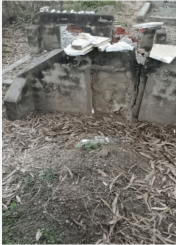
Debris of damaged headstones
